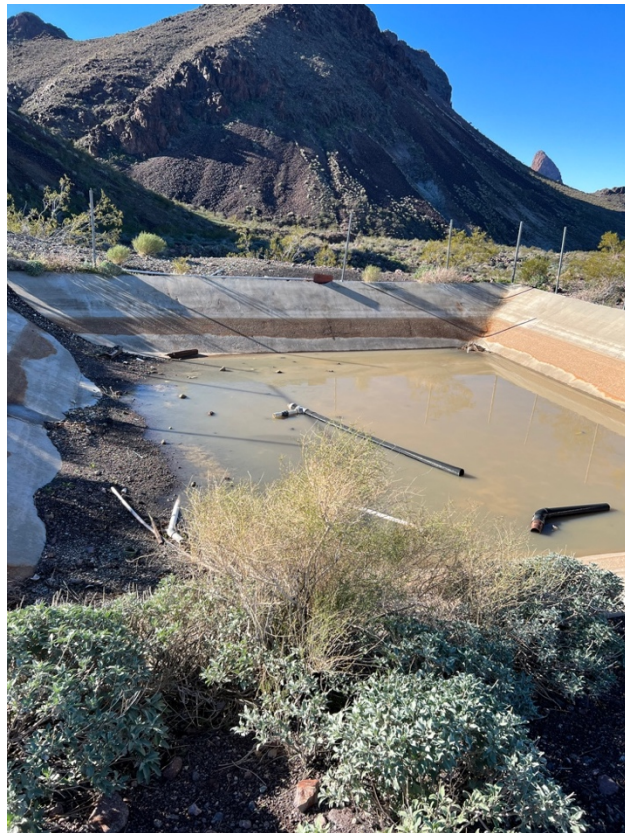
Figure 3.1: Abandoned Sedimentation Pond (photo credit: Frankie Martinez)
