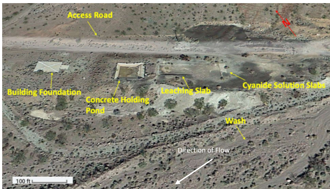
Figure 1.4: Current Site Condition [1]
